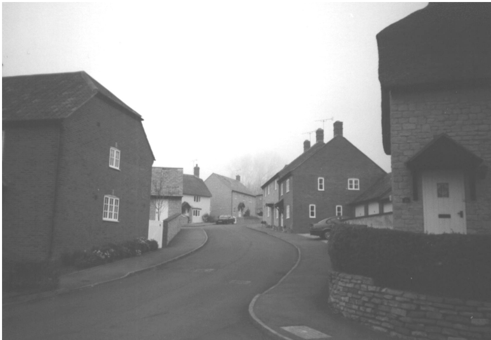
Figure 8.2 New housing in the village of Burton Bradstock, Dorset, built in the local vernacular using reconstituted stone
