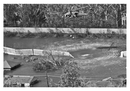
Failure of the levee along the London Avenue Canal, along with breaches in the 17th Street and Industrial canals, led to widespread flooding in New Orleans. The back side of Hurricane Katrina's storm surge pushed water down the narrow canals. When the walls collapsed, water quickly covered 80 percent of the city.
